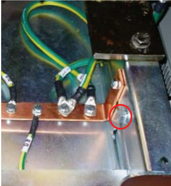
Figure 11-4 : Connection of earth wire protection (PE)
